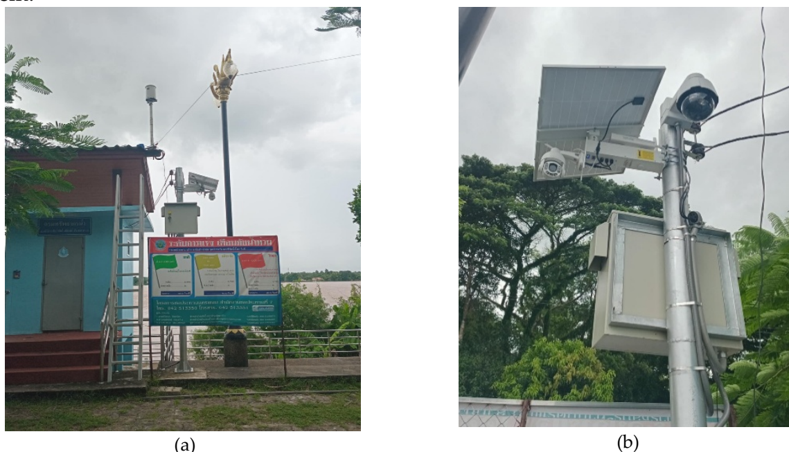
Figure 5 Installation of Mekong River water level monitoring system. (a) Location of water level monitoring station and (b) installation of the system.
